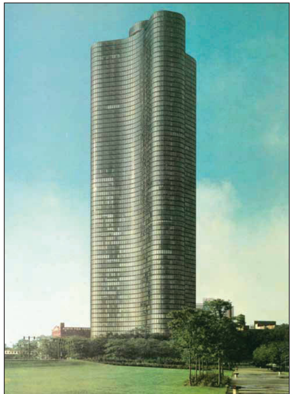
The 70-story glass-curtained Lake Point Tower is one of the most widely recognized Chicago landmarks. The residential high-rise, located at 505 N. Lake Shore Drive, was completed in 1968 and 20 years later converted to condominiums by American Invsco.
